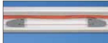
TGFSB installed in TG-70 Raceway
