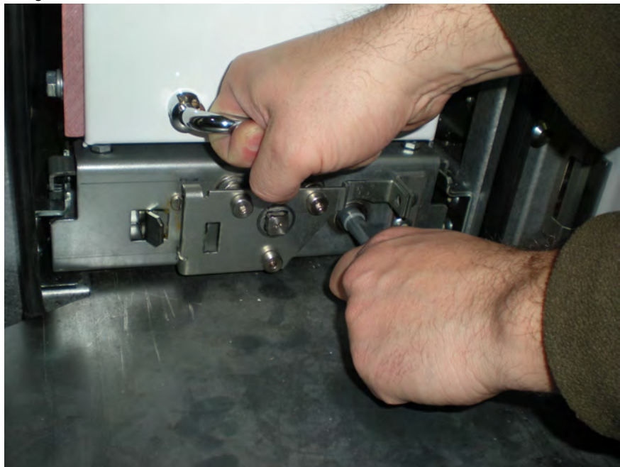
Figure 20 - Contactor Cart Removal Handle
