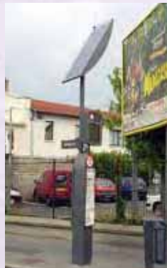
Photovoltaic system at Villeurbanne, France
