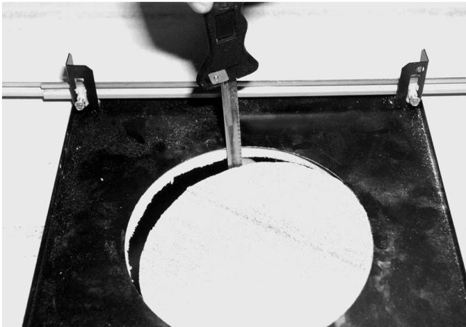
**Figure 3.2** Cut Hole in Ceiling Tile
