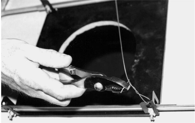
**Figure 3.4** Secure Bracket Assembly
